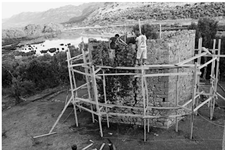
Fig. 9 Restoration/ consolidation work on the apse wall
