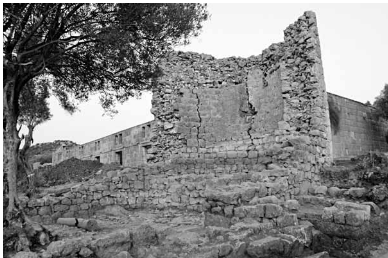
Fig. 11 General view from the north after the excavations
